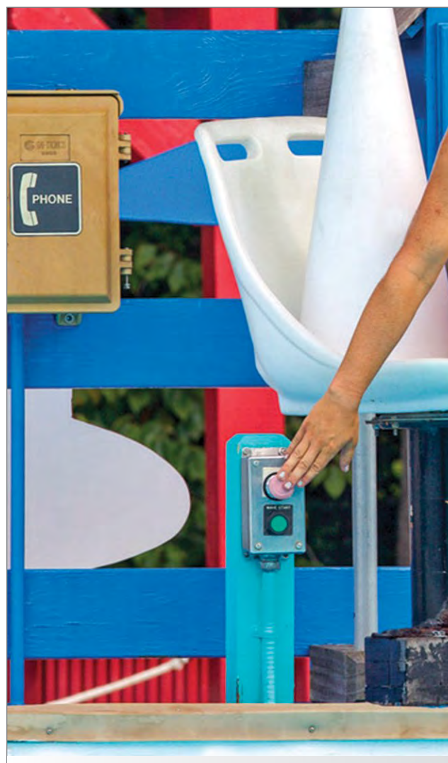
Figure 4-14 | An emergency stop (E-stop) button can be pressed to turn off the waves in a wave pool when a rescue is required.
